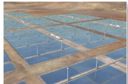
Multi-plant CSP Farm
